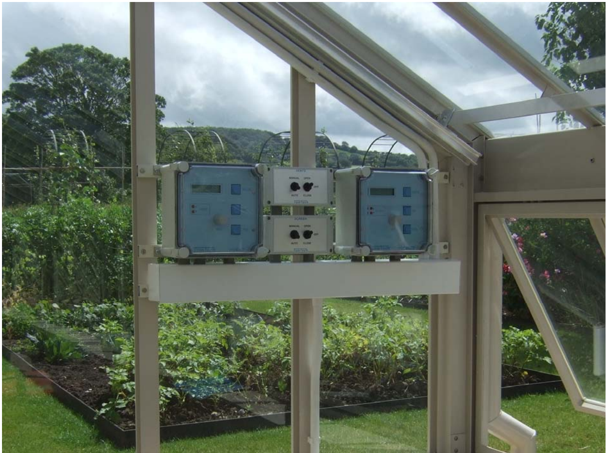
MicroVent and Micro Screen Installation
